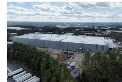
An aerial photograph showing the construction site of a DataBank data center in Atlanta. PHOTO: HYOSUB SHIN/THE ATLANTA JOURNAL-CONSTITUTION/ZUMA PRESS
