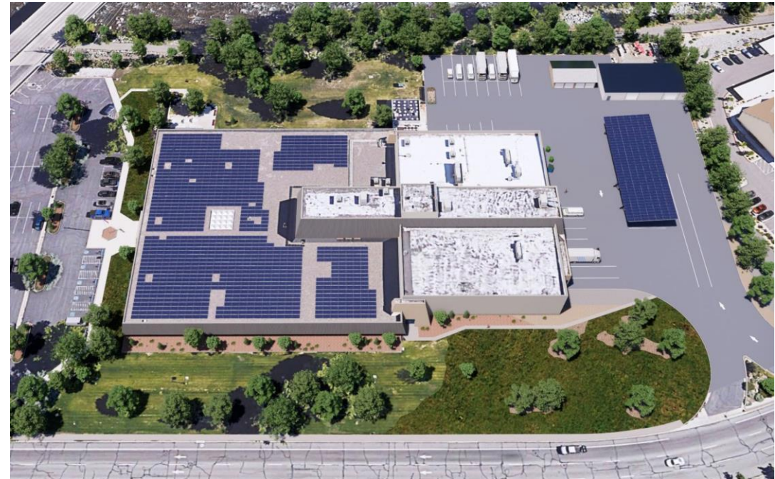
Pictured: Proposed microgrid for City of Reno Public Safety Center that was awarded FEMA Building Resilient Infrastructure and Communities (BRIC) funding (Source: Ameresco)
